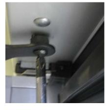
Figure 11 Remove Hold-Open Bolt
