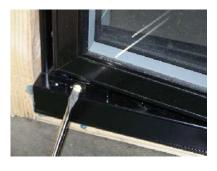
Figure 10 Release TorqueMaster Tension
