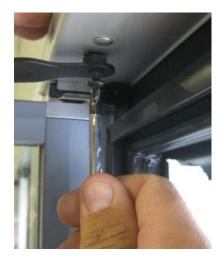
Figure 9 Tighten Hold-Open Bolt
