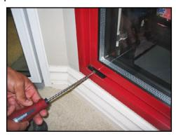
2. Open the door to access the hold-open device, then loosen and remove the hold-open detent bolt, using a 7/16" hand wrench.
