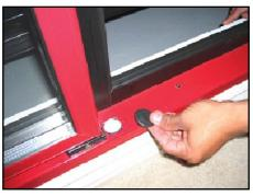
4. Place the Torquemaster on the newly opened mounting pocket in the frame, with the hollowed end of the Torquemaster towards the frame.
