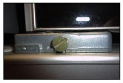
Release Torquemaster Tension
