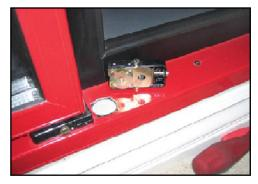
6. Turn the mounting set-screw clockwise to engage the mounting mechanism underneath the frame lining, then confirm that the Torquemaster is securely mounted.
