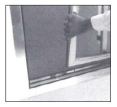
6. Note that Roller cage does not screw into bottom of door.
