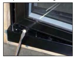
2. On Models 401 & 403: Open door and lock into hold-open position. Using a flathead screwdriver, go to the top and remove the hold-open bolt from the frame by turning the bolt hex head counter-clockwise.
