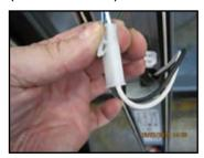
Disconnect wire connector at top of driver (black & white)
